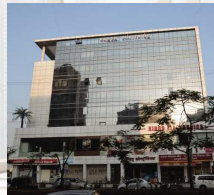
Completed - Parth Solitaire, Kalambohi, Navi Mumbai
